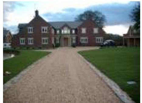
A prestige Cheshire Installation of Nidagravel using reclaimed stone setts and 10mm golden gravel
